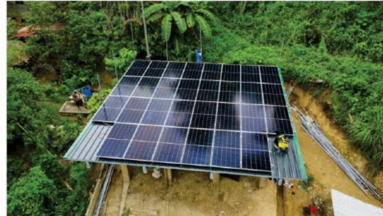
SOLAR WATER SYSTEM PHASE 1 (CONSTRUCTION PROGRESS)
